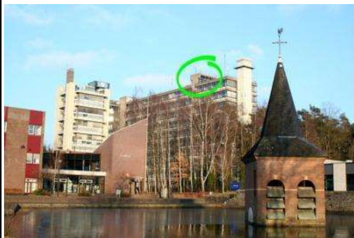
Figure a- the building in which the system is located
